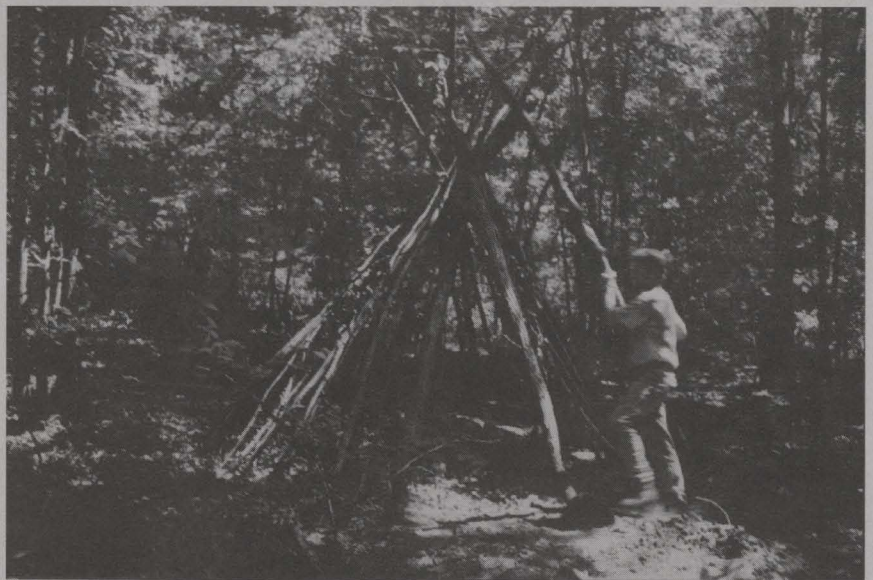
Beginning the structure by laying poles against a central tripod.
