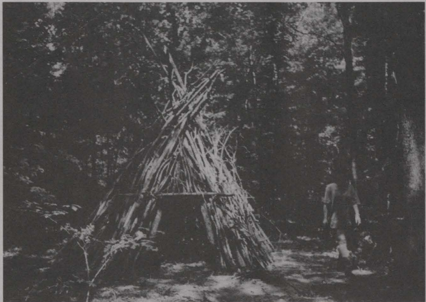
Burned sections are stacked randomly to fill in voids and a lintel is lashed in place to form the door.
