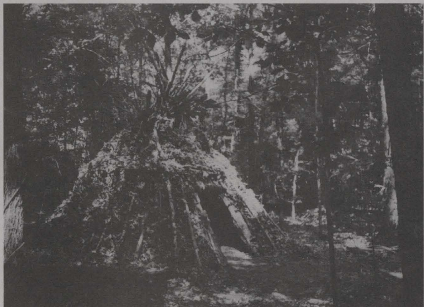
The entire structure is covered with leaf litter, bark, and more deadfall timber that keeps the leaves in place.
